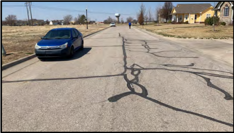
TIGHT or SEALED CRACKING
