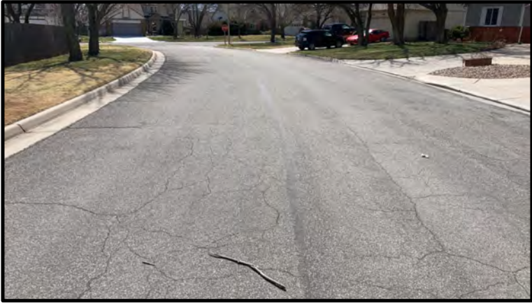
TIGHT or SEALED CRACKING
