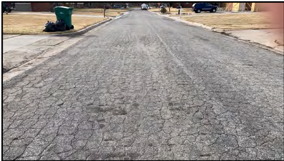
ALLIGATOR CRACKING
